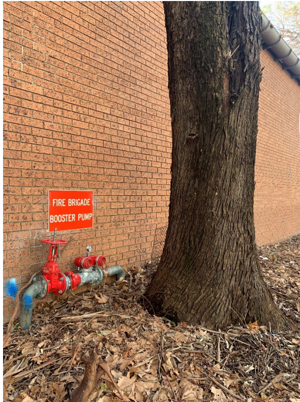
Figure 22 - Tree 25 proximity to existing building
